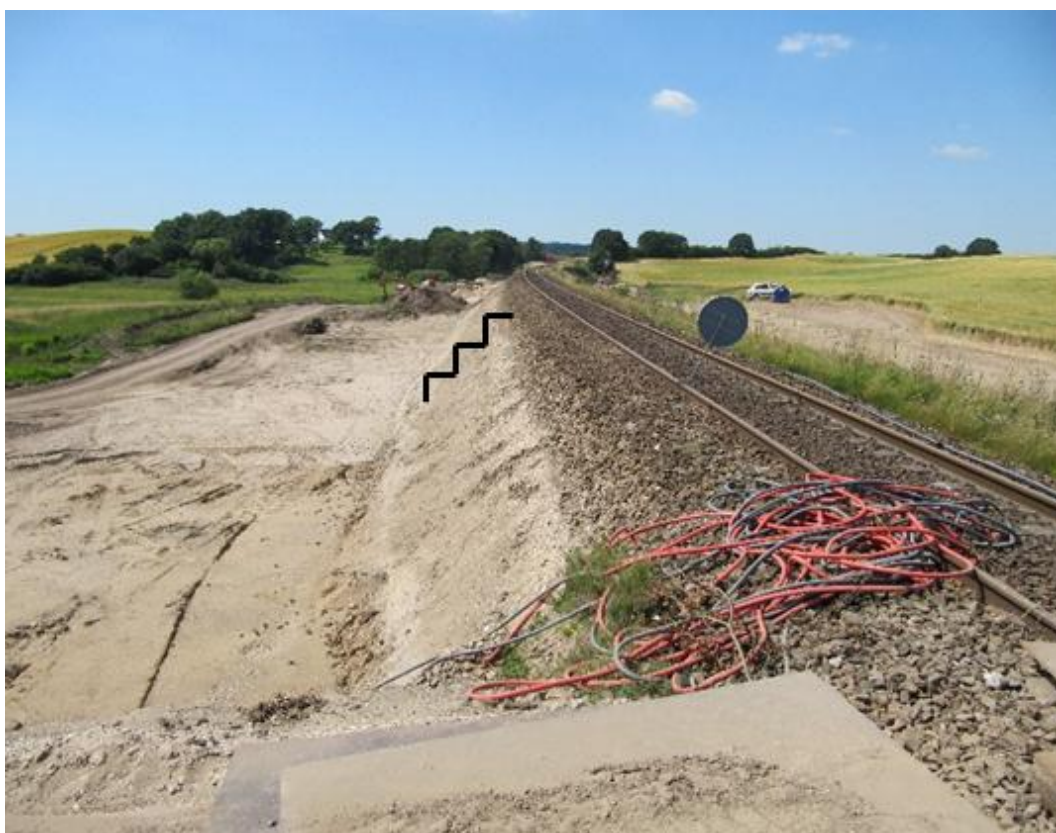
Figur 9.1.8. Trappeafgravning.
