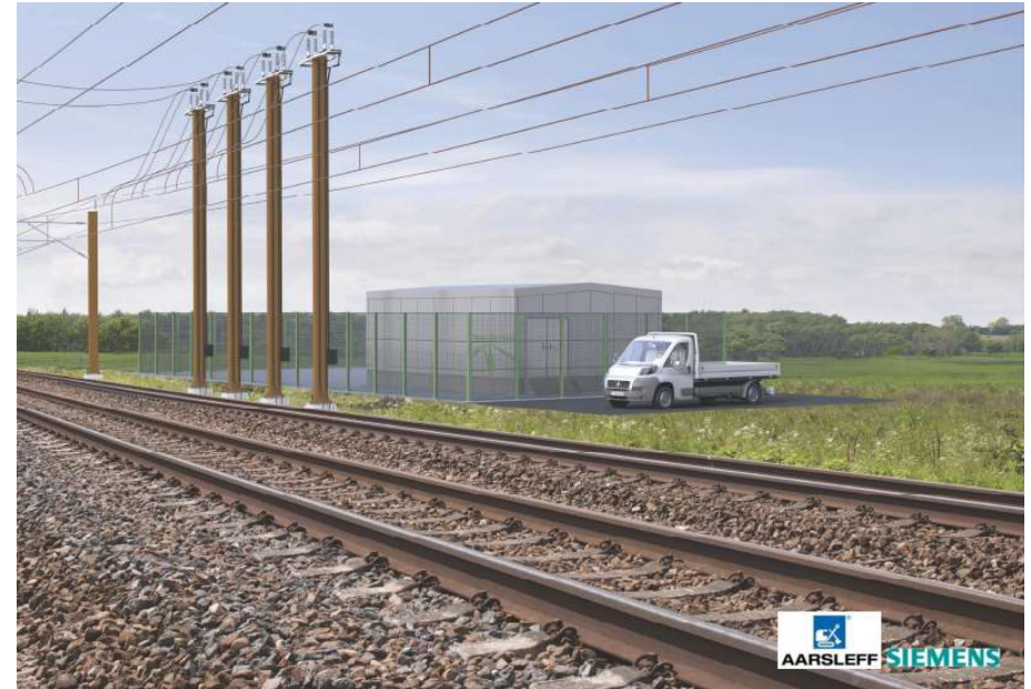
Autotransformerstation
